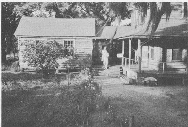
Fig. 22.--WPA community reading room at Murrell's Inlet (Georgetown County).
